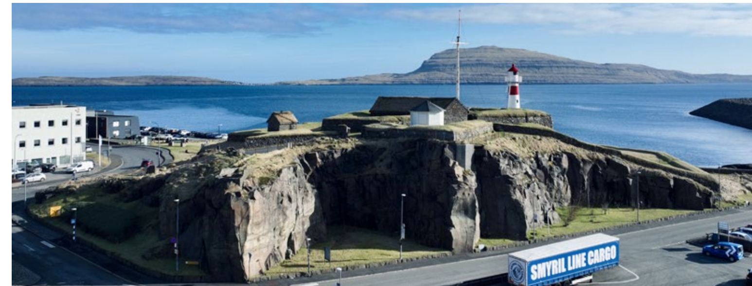
The view from the soon-to-come Roof Top Café before the transformation of the area. Viewing eastward.
